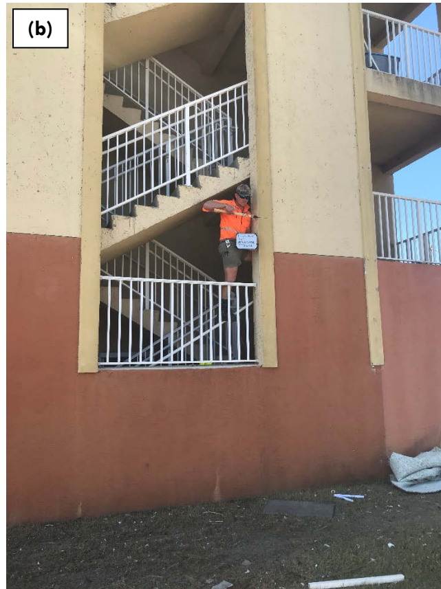
Figure 7. (a) USGS high water mark survey of a seed line within the stairwell of a vacation rental building in Mexico Beach, Florida. (b) Measurement of the height of the seed line from ground level on the exterior of the building. Images courtesy of the USGS.
